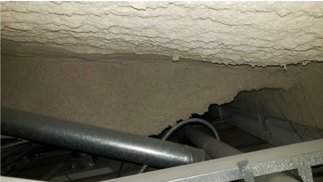
Figure 68 - Fire protection over roof joist framing
