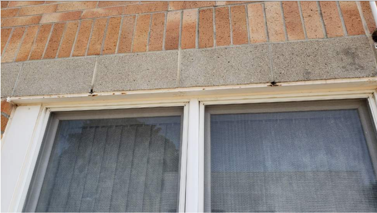
Figure 93 - Corrosion at lintel on north wall
