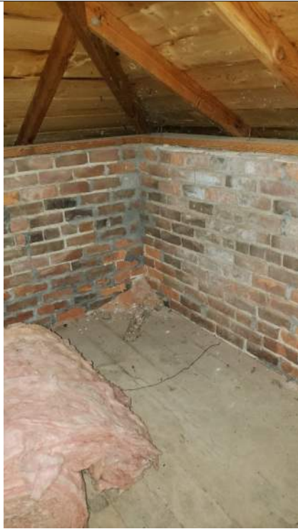
Figure 7 - Stair tower walls at attic showing brick degradation
