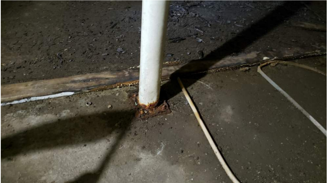
Figure 55 - Corroded column base at cellar storage area
