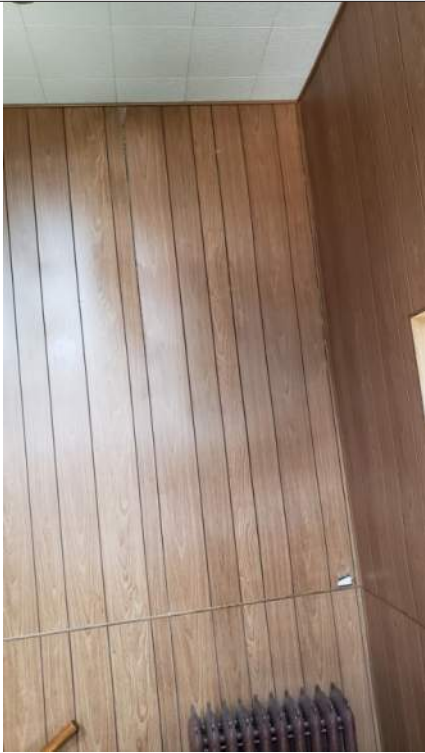
Figure 45 - Warping of finishes at stair tower
