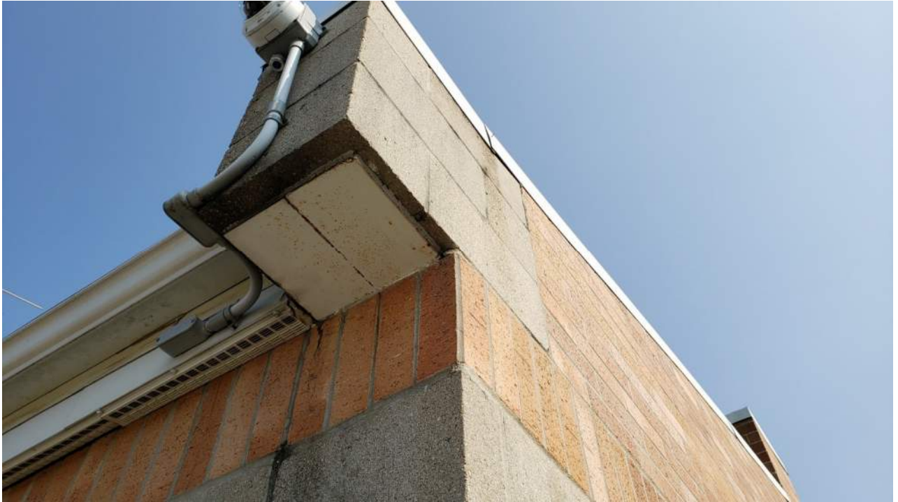
Figure 83 - Corrosion at masonry support
