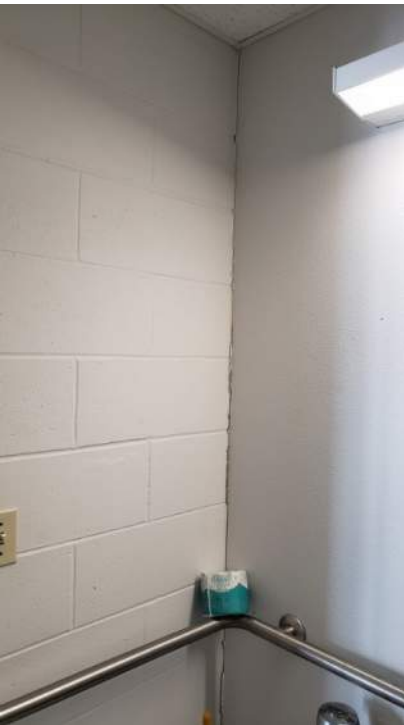
Figure 63 - Wall crack at rest room
