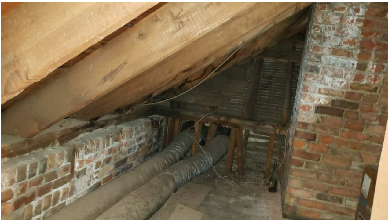
Figure 72 - Roof framing at west wall showing efflorescence
