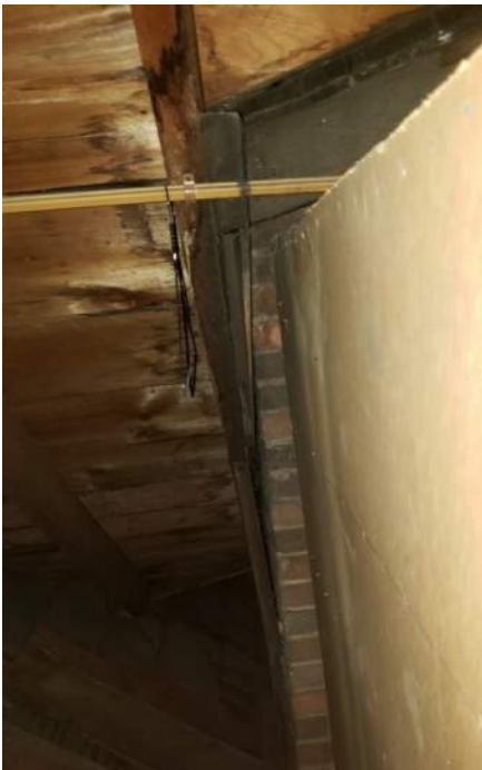
Figure 37 - Roof framing north of stair tower pushed away from wall
