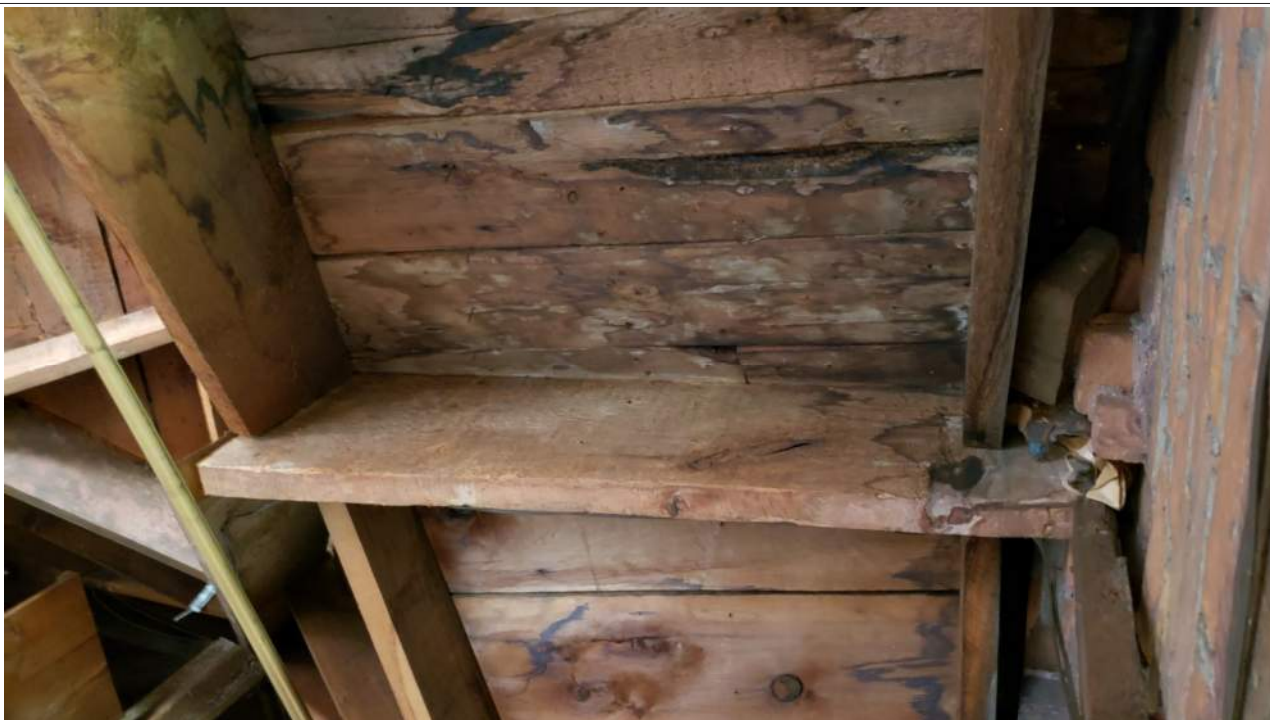
Figure 11 - Water infiltration at deflected framing member
