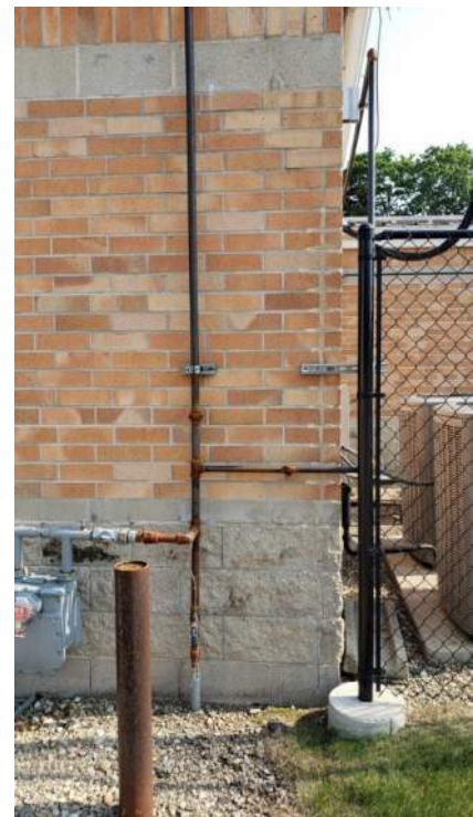
Figure 82 - Previously repaired masonry at exterior
