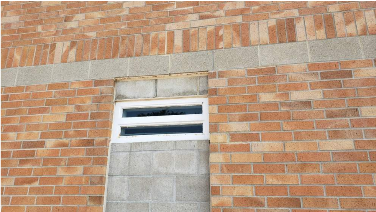
Figure 85 - Corrosion at steel lintel
