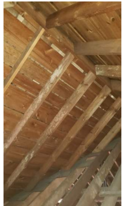
Figure 28 - Roof framing - south gable framing into main ridge
