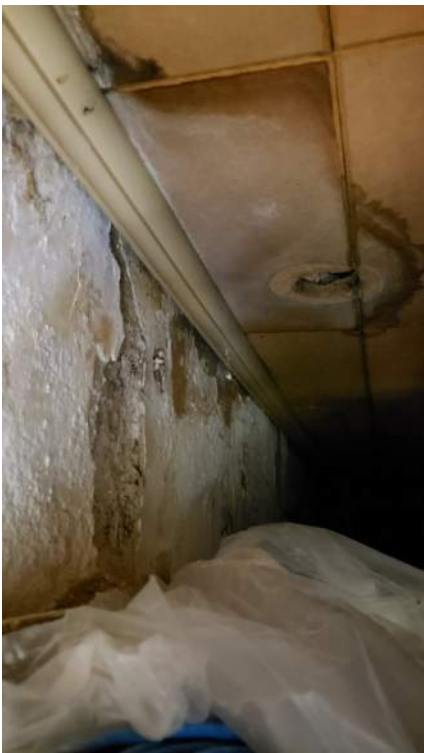
Figure 47 - Water infiltration at office ceiling adjacent to stair tower
