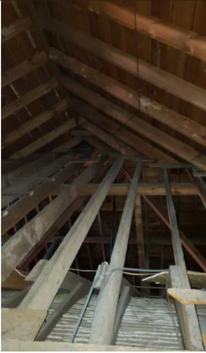
Figure 25 - Roof framing over courtroom arched ceiling where south gable joins
