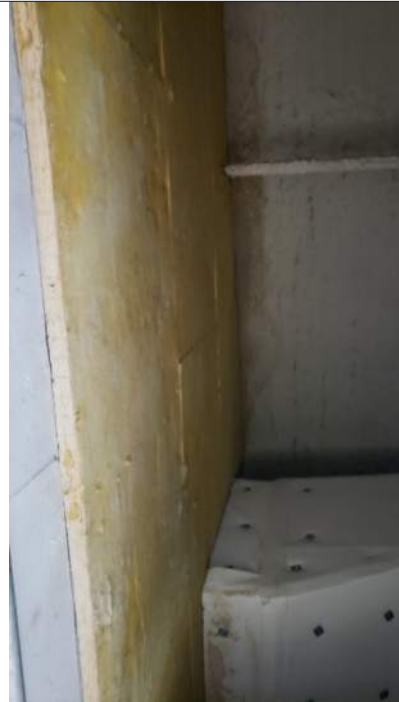
Figure 62 - Water staining above offices on south side
