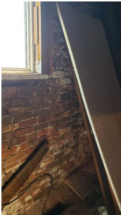
Figure 9 - Wall at south gable showing some cracking and efflorescence
