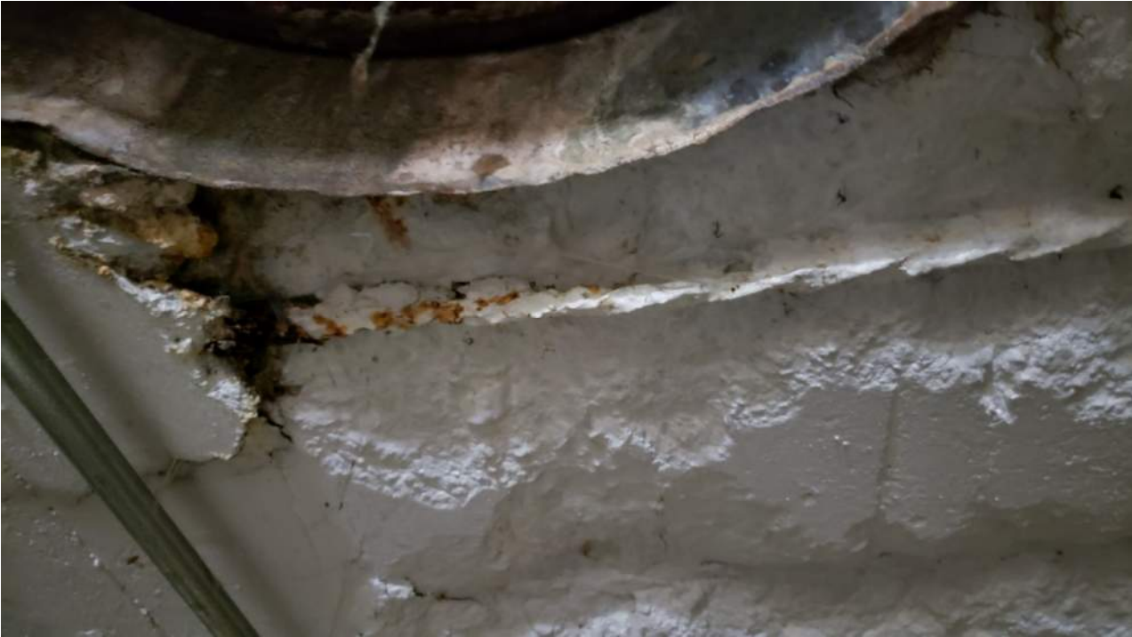
Figure 57 - Spalled concrete with exposed and corroding reinforcement
