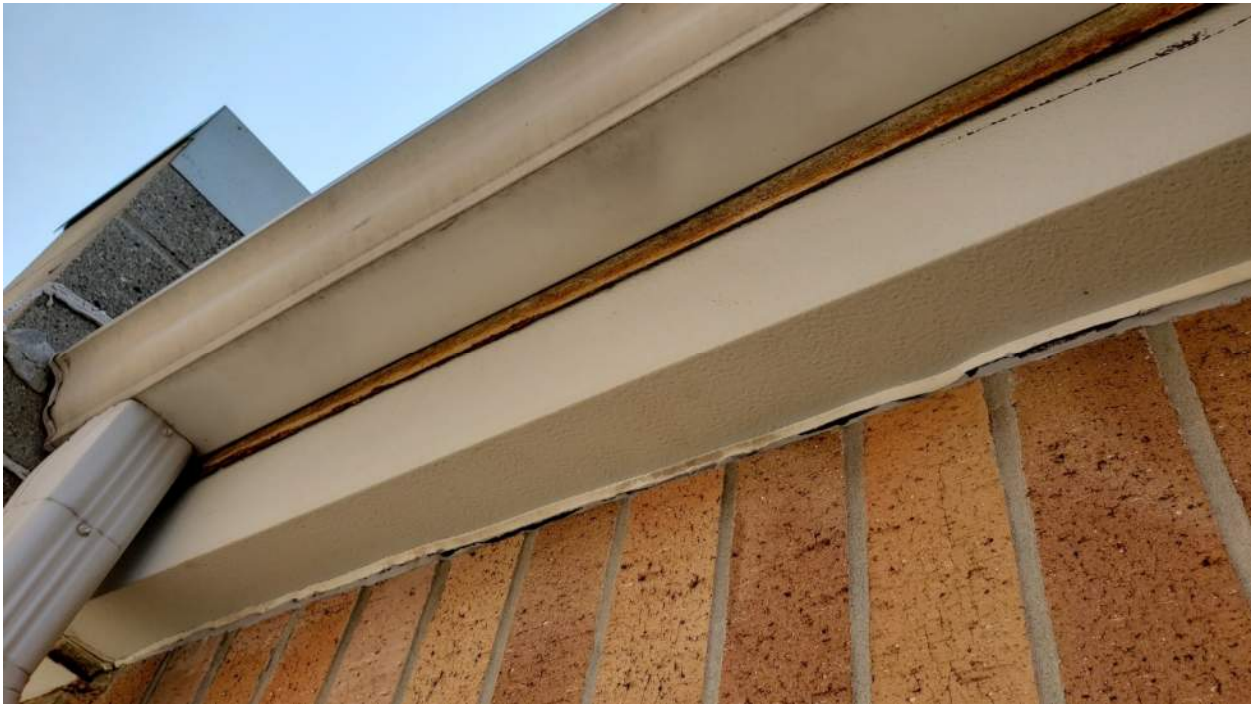
Figure 60 - Loose caulk adjacent to the southeast entrance
