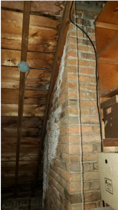
Figure 9 - Roof framing at chimney showing water damage and brick efflorescence
