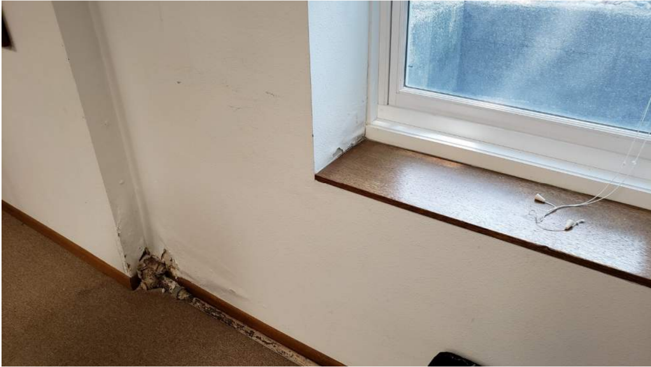
Figure 53 - Water damage at southwest office, lower floor
