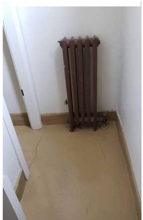
Figure 38 - Slab crack at 1938 addition rest room
