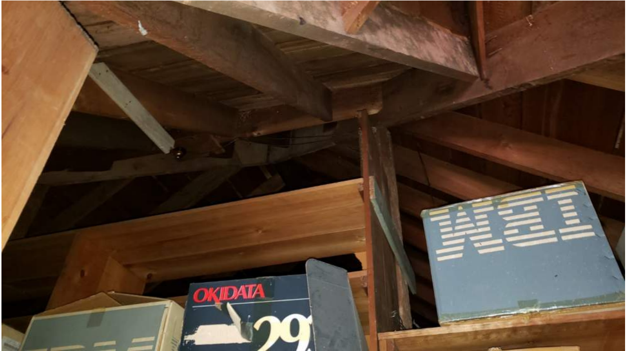
Figure 5- Roof framing at south facing roof
