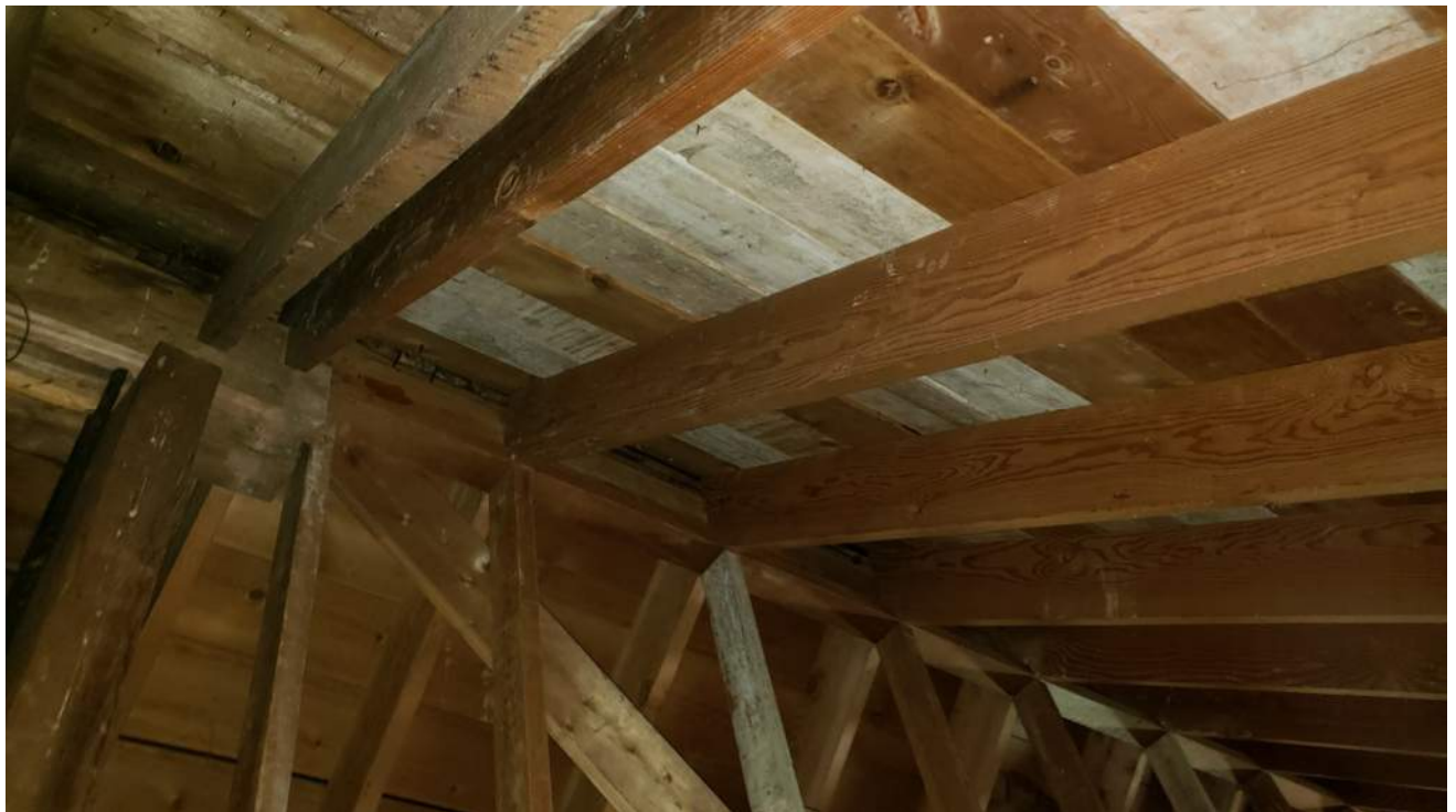
Figure 32 - Roof framing at 1938/1893 connection
