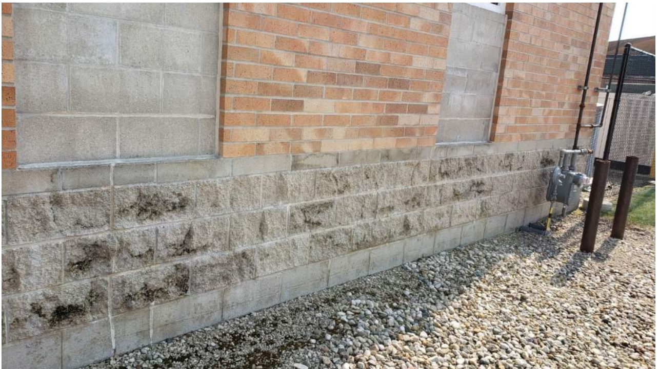
Figure 84 - Previously repaired cracked exterior masonry
