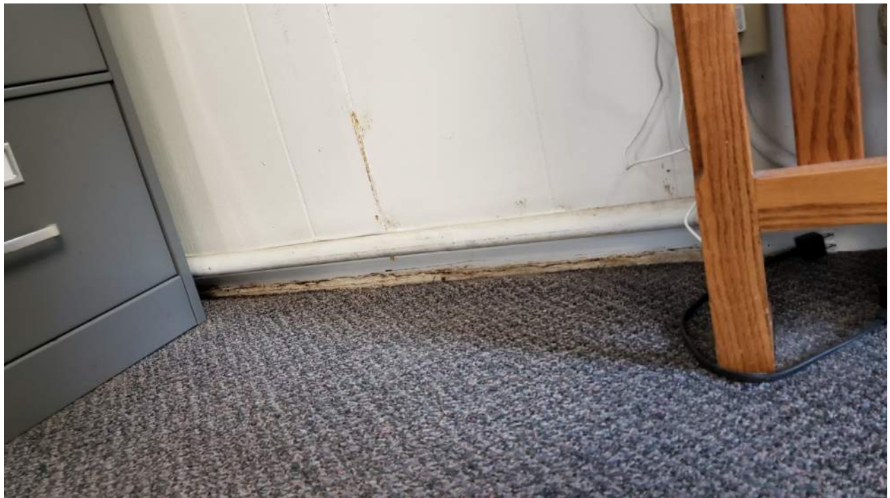
Figure 52 - Corrosion at floor immediately below window well location
