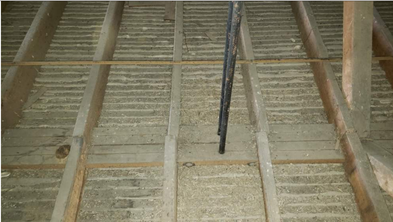
Figure 29 - Roof truss bottom chord over courtroom with arch framing
