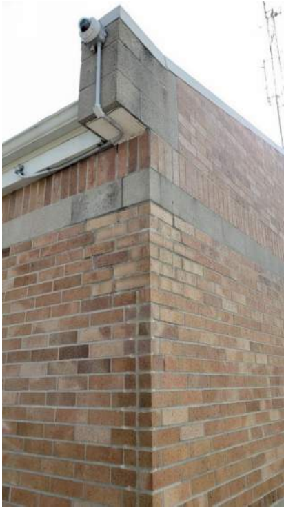
Figure 79 - Previously repaired masonry at exterior
