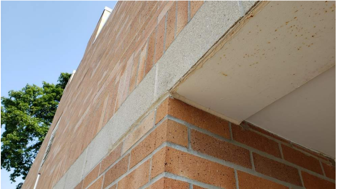
Figure 87 - Corrosion at lintel
