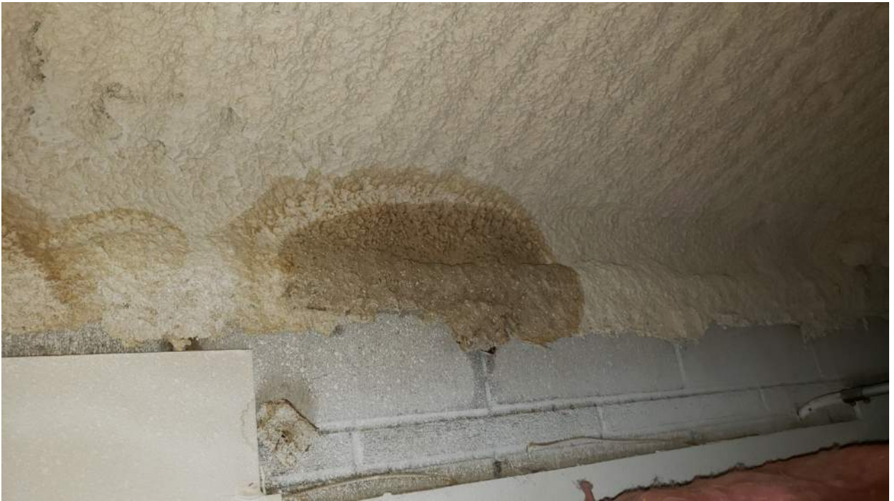
Figure 69 - Water intrusion near southwest corner
