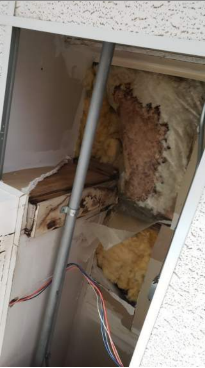
Figure 61 - Water intrusion at northeast entrance
