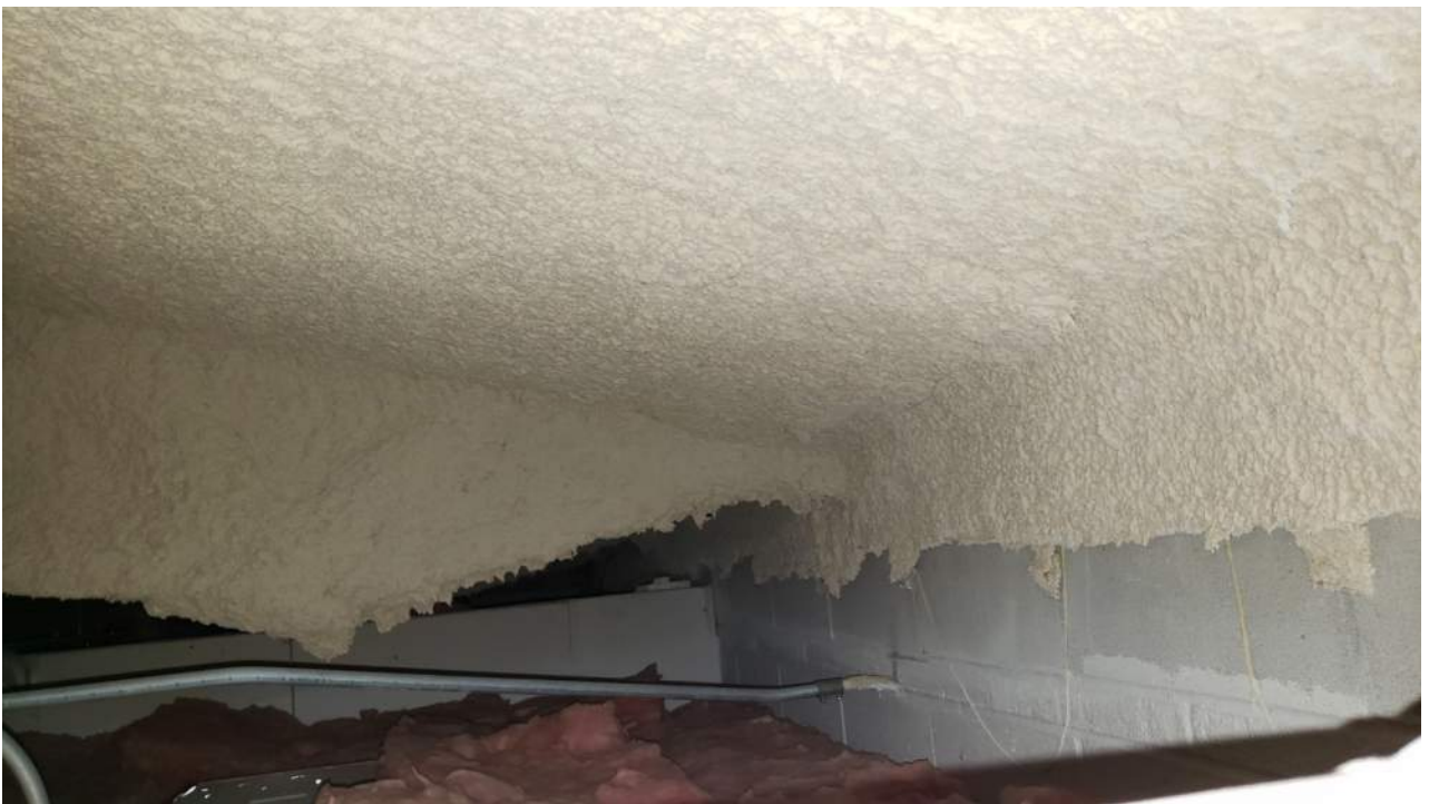
Figure 70 - Fire protection over steel joist framing
