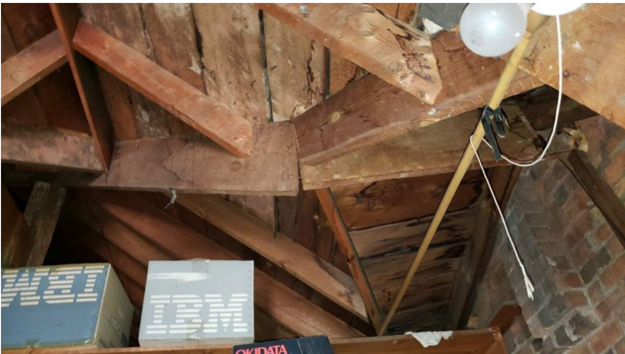
Figure 4- Roof framing west of stair tower showing water infiltration and connection failure
