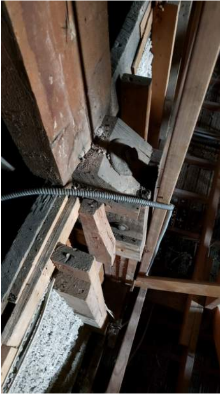
Figure 35 - Main roof truss bearing at 1893/1938 connection
