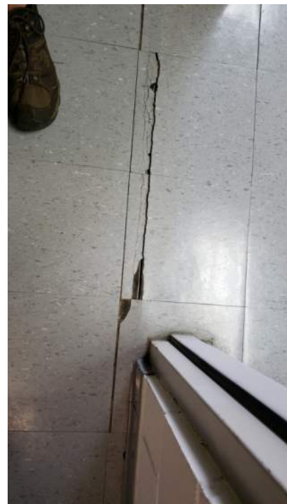
Figure 64 - Floor crack at rest room
