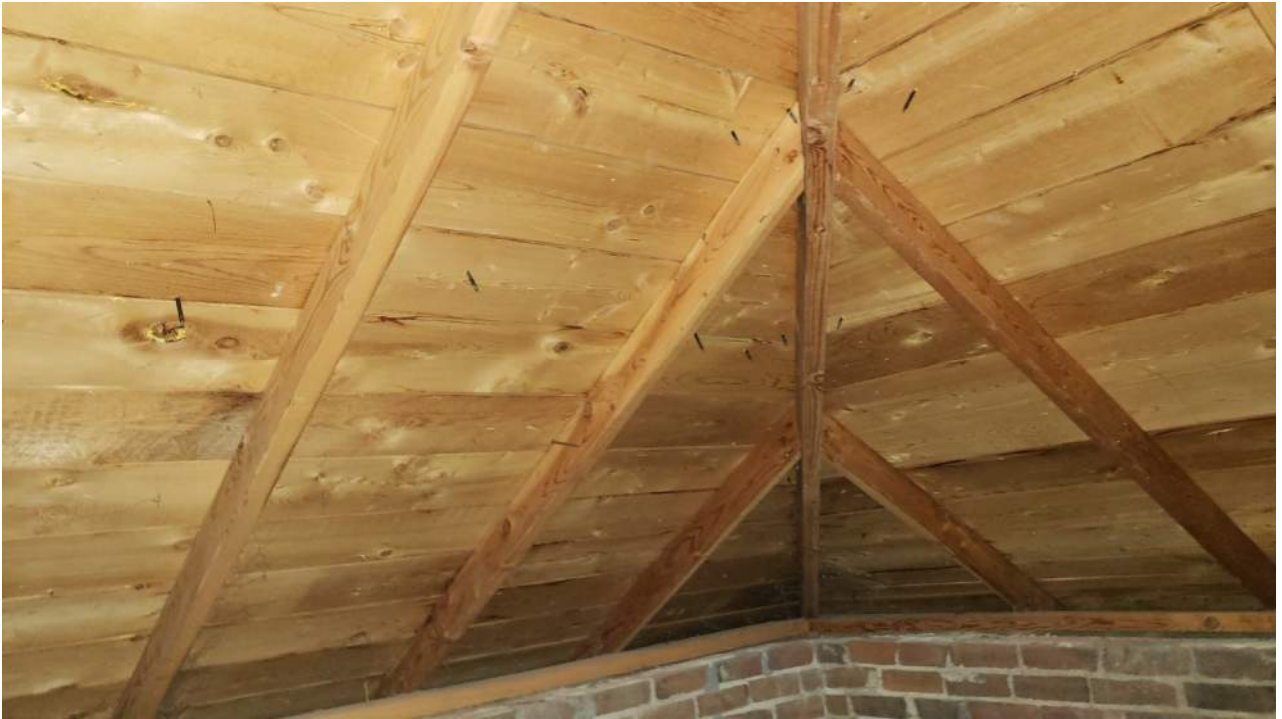
Figure 1- Framing at stair tower roof
