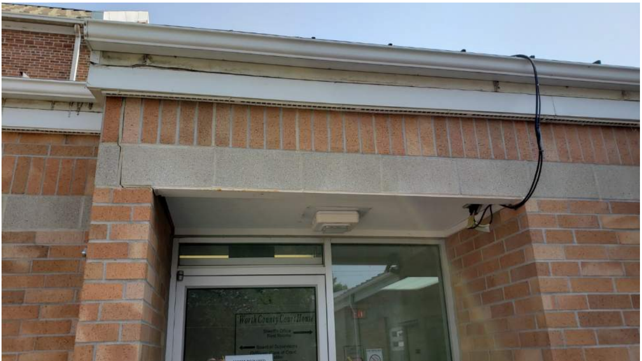
Figure 92 - Crack at lintel bearing at northwest entrance
