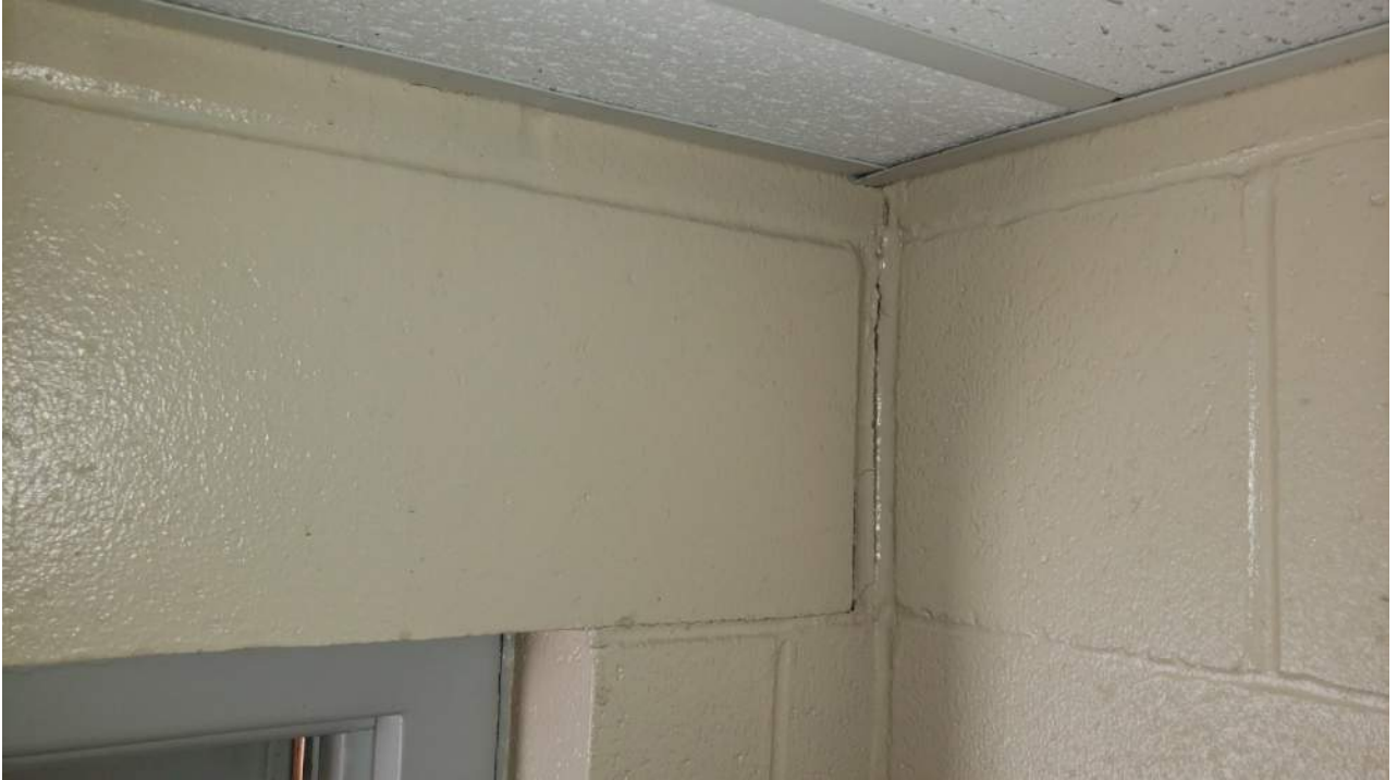
Figure 77 - Cracking at southwest entry lintel
