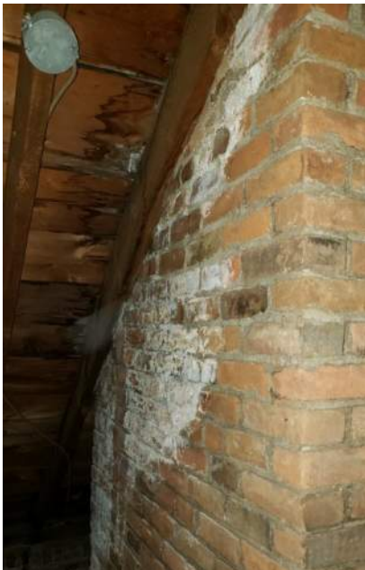
Figure 15 - Water infiltration and efflorescence at chimney
