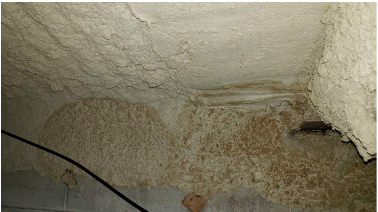
Figure 66 - Discoloration of fireproofing at southeast corner
