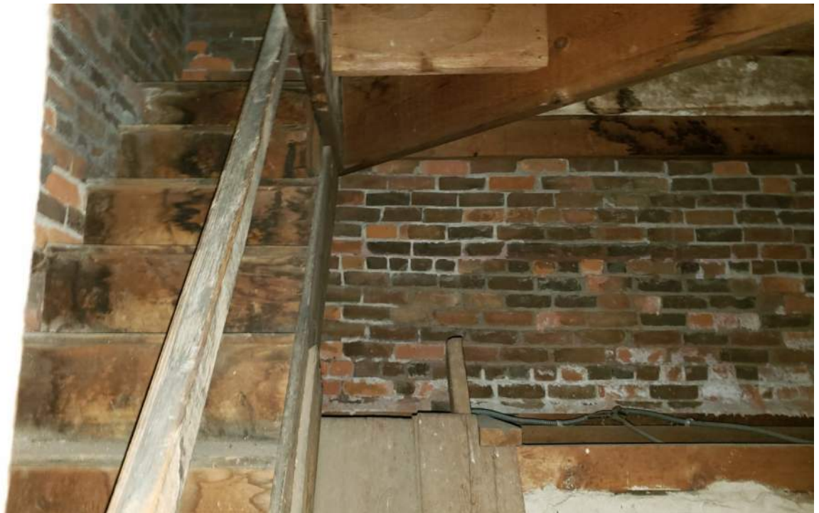
Figure 2- Stairs up to attic and stair tower wall degradation
