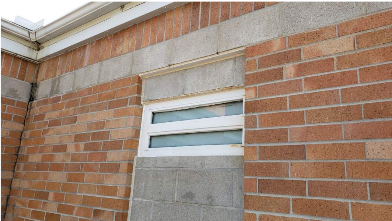
Figure 86 - Corrosion at steel lintel, moisture accumulation in corner
