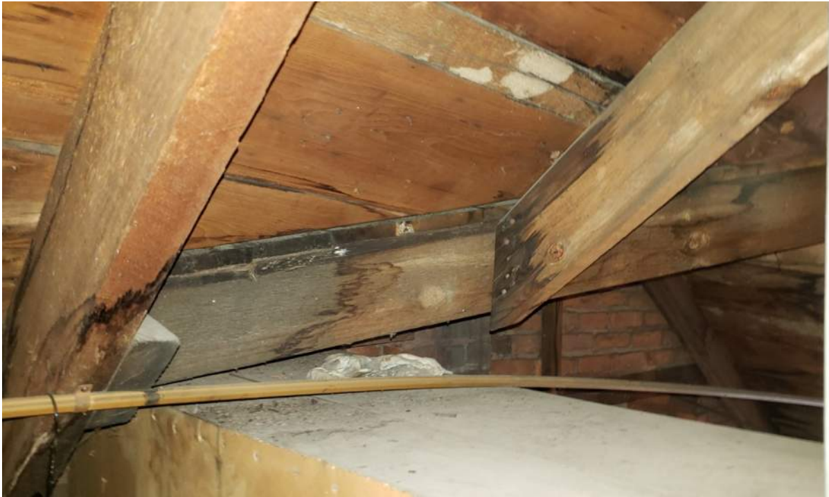
Figure 41 - Weathered roof framing adjacent to the northwest corner of stair tower
