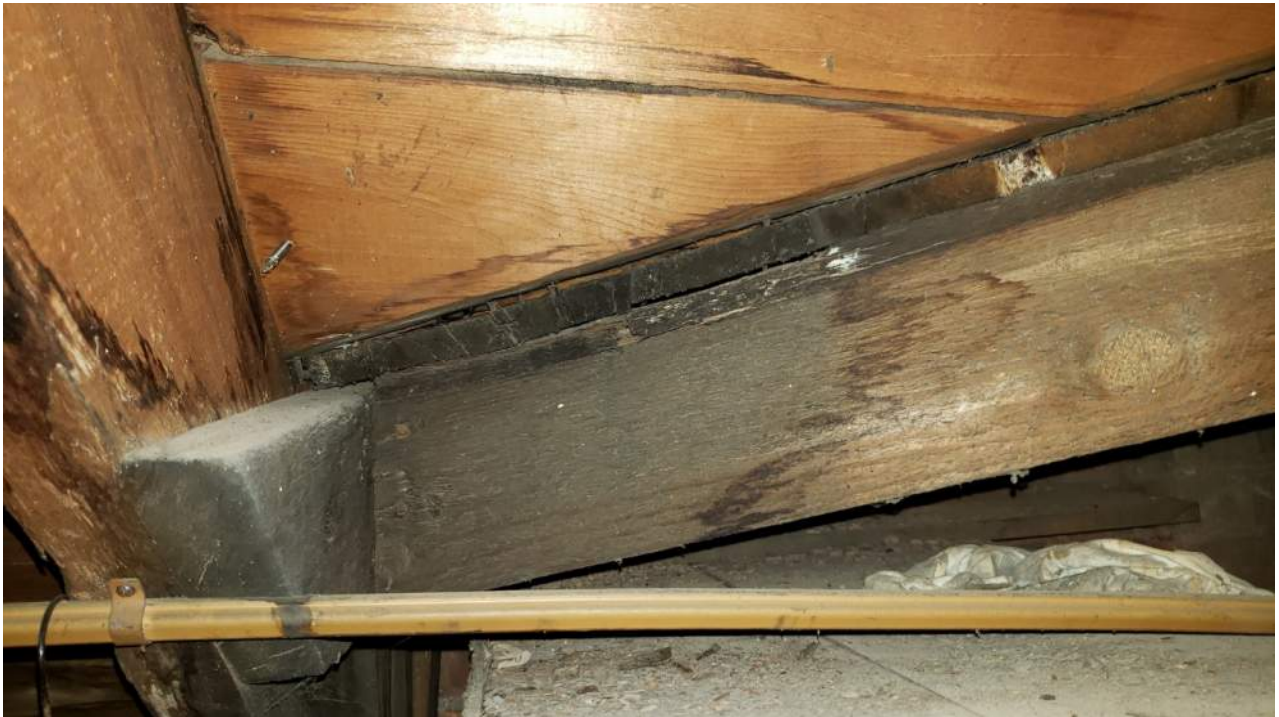
Figure 42 - Water damaged roof framing adjacent to northwest corner of stair tower
