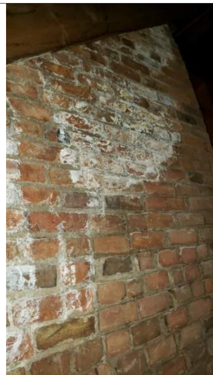
Figure 18 - Chimney showing significant efflorescence
