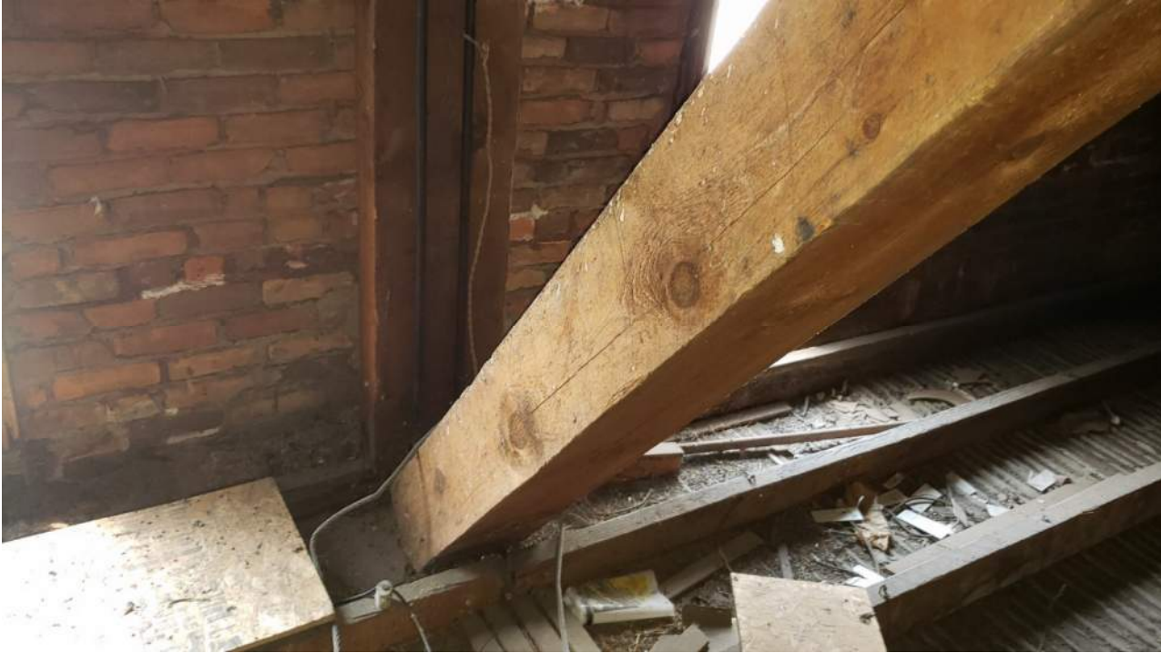
Figure 39 - Main roof truss bearing at west wall
