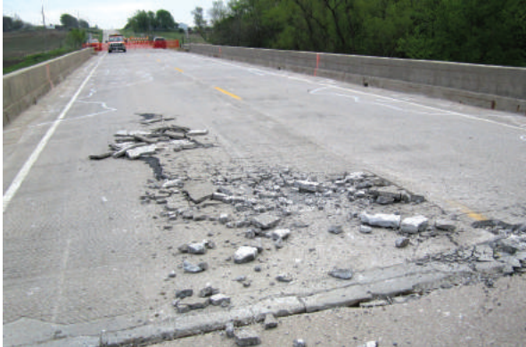
Temporary closure to traffic.
